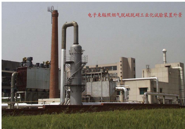
Figure 8: pilot plant constructed by CAEP for removing SO 2 and NO x in Mianyang, Sichuan
